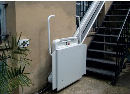
Niche Inclined Platform Lifts are designed for straight stairways, and their compact folded platforms provide a smooth ride for wheelchair users. Their fully automatic operation makes them safe and easy for passengers to utilise, with no special training or requirements necessary to operate them.
