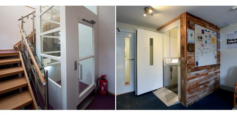
The Niche internal platform lifts provide safe, efficient and smooth vertical travel up to 9 metres (6 floors). With their free-standing and self-supporting structure (requires anchoring to the building), and options for no pit and no motor room, the platform lifts are both quick and easy to install.
